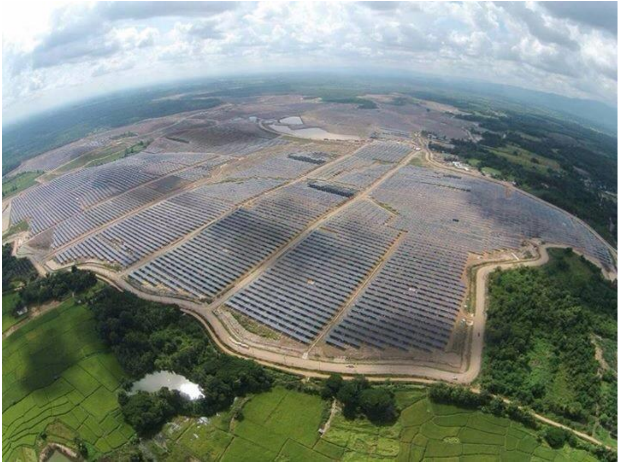
Figure BangPa In Solar Farm with the capacity of 44MW with NanoPV group system design and engineering, 2014
