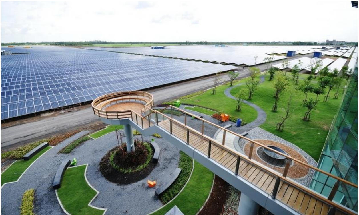
Solar Farm control room with viewing stage and a BIPV building
