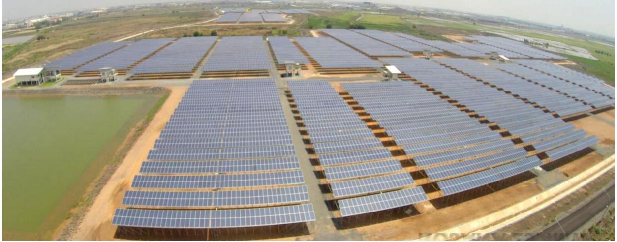
Rojana solar farm with the capacity of 29.4MW: NanoPV group system and engineering
