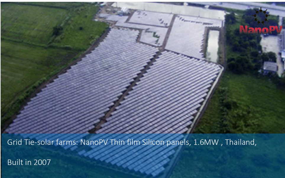
Utility Scale solar farms: thin Film Si using NanoPV technologies, 1.26MW, Thailand, Built in 2007
