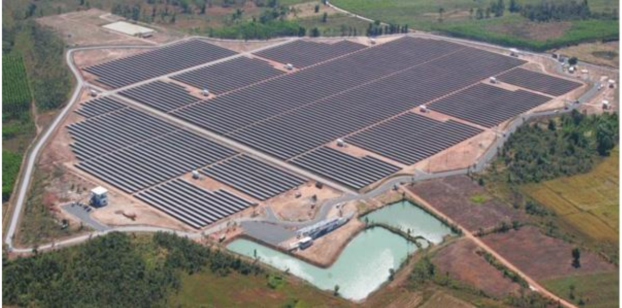
Prachin buri Solar Farm, 25MW, designed and engineered by NanoPV group, 2014.
